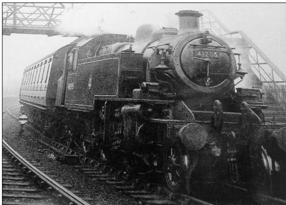
'Push-and-pull' service with Ivatt 2-6-2T No.41285 standing at Earlestown. Note the vacuum valves fitted to the sides of the smokebox. Photographer : Unknown
